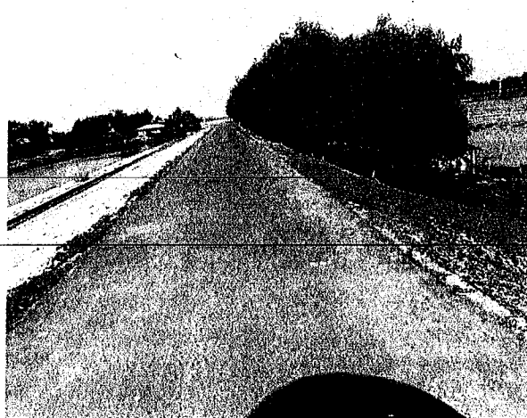
Figure: Embankment as Upgraded by CEIP-1
