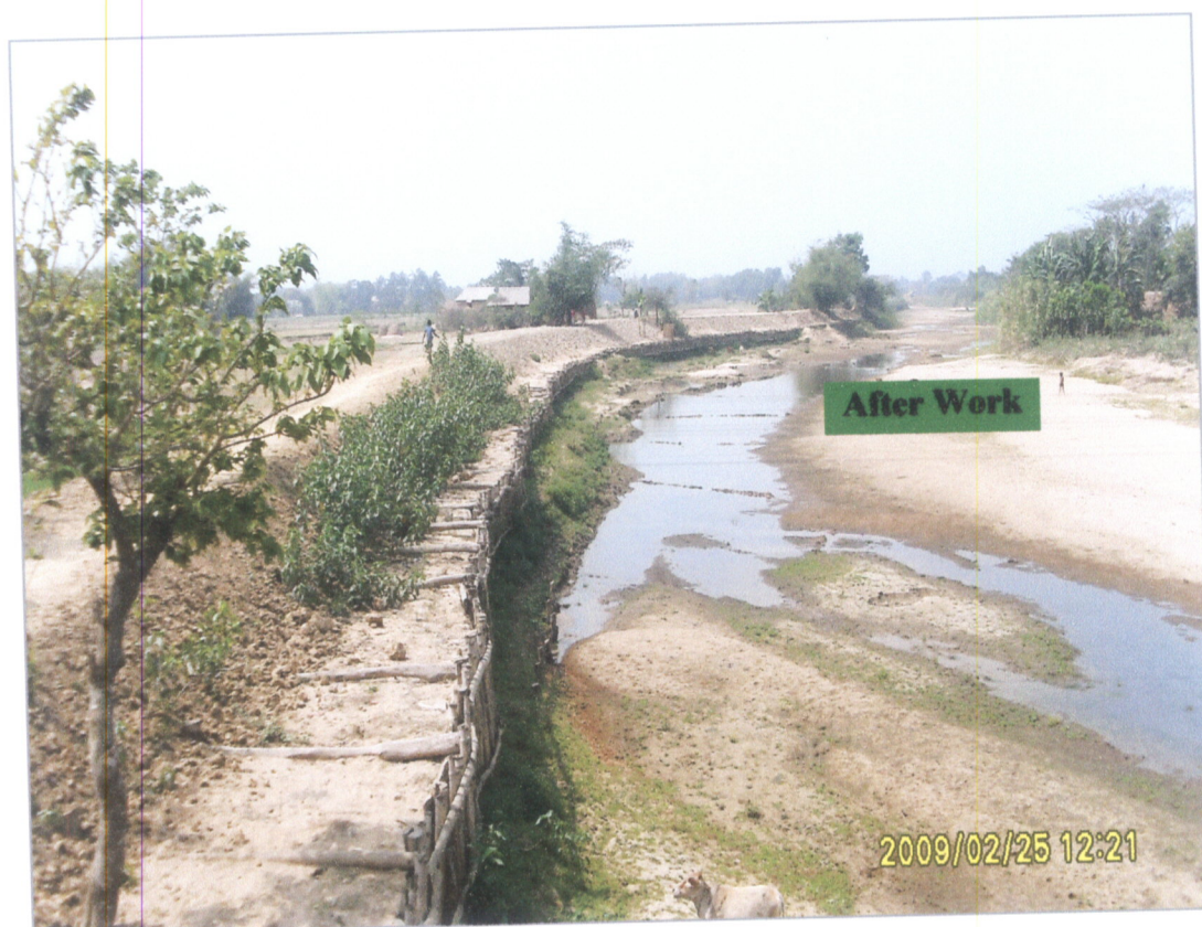
Contract No. BWDB-HAB-01: Sonai River, Left Bank, Upa: Madhubpur, Dist: Habiganj.
