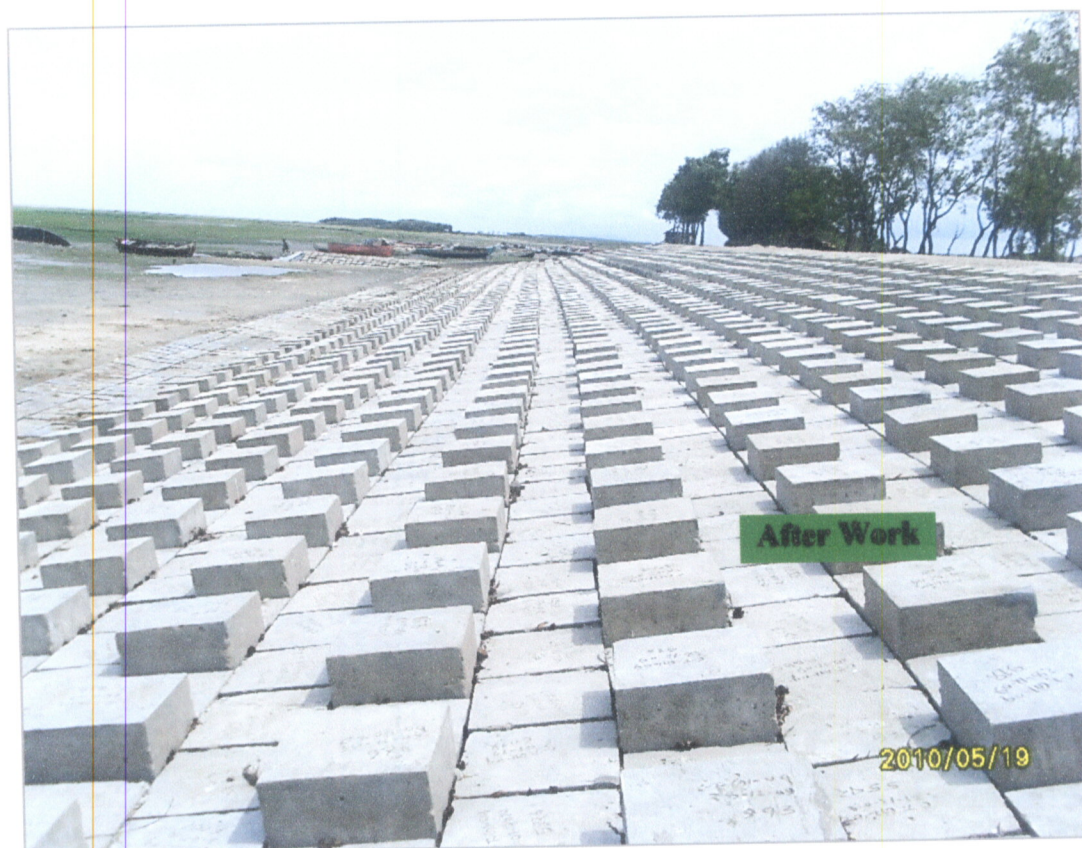
Contract No. BWDB-CTGI-04: Left bank of Sandwip Channel at Anandabazar, Upazilla: Chittagong Sadar, District: Chittagong.
