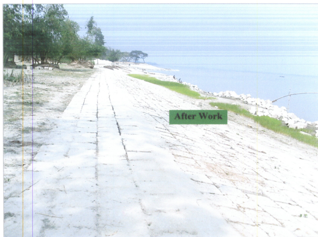
Contract No. BWDB-BOG-05, 06, 07& 08: On the right bank of Jamuna River at Talukdarpara, Upazilla-,Sariakandi, District- Bogra.
