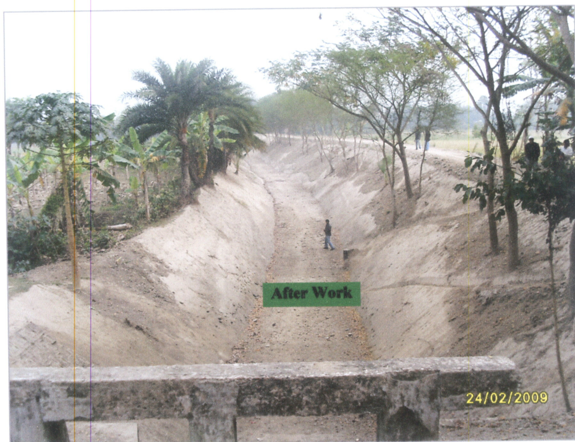
Contract No. BWDB-RAJ-02: Re-excavation of Moharajpur Irrigation Canal (SWZ-09), Upazila: Faridpur Sadar, District: Faridpur
