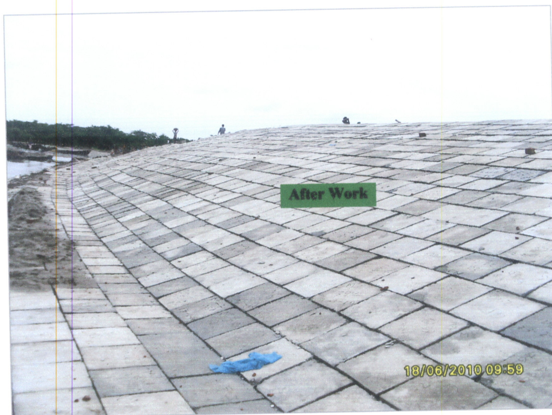
Contract No. BWDB-MAD-07: Left Bank of Arial Khan river at Haji Shariatulla Bridge, Upazila: Shibchar, District: Madaripur.
