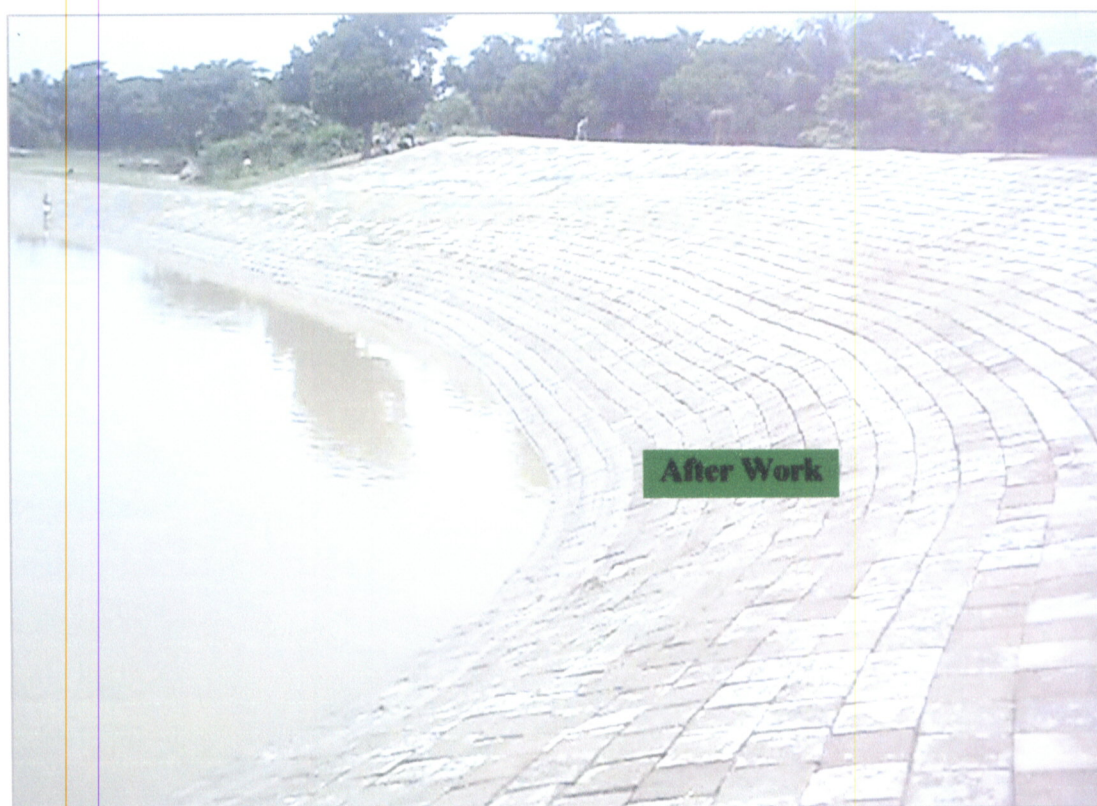
Contract No. BWDB-GUM-02: Right bank of Gumti river at Chandpur, Upazilla : Devidwar, District: Comilla.
