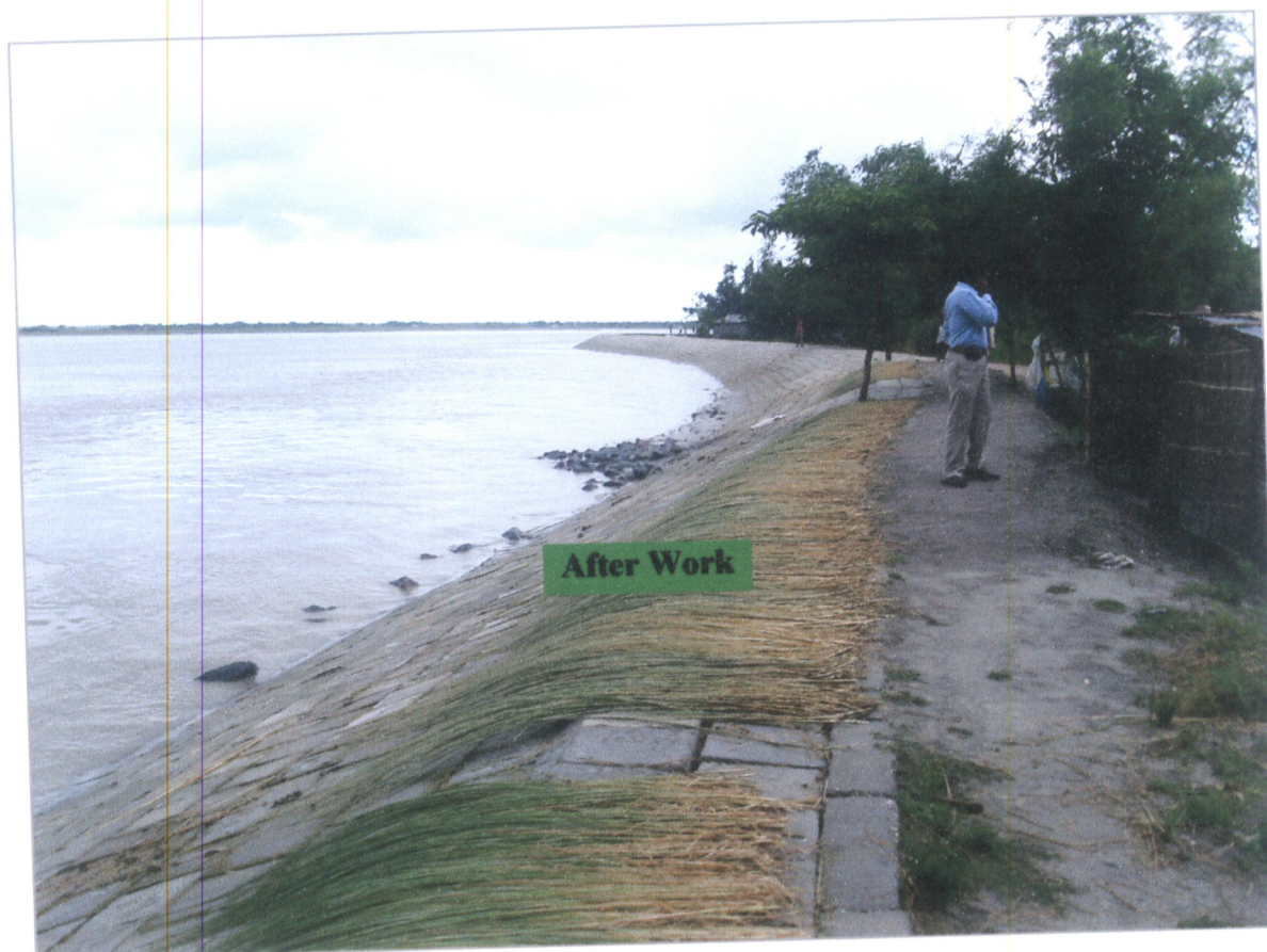
Contract No. BWDB-RAN-07: Right bank of Teesta River at Gannarpar, Upazilla-Gongachara, District- Rangpur.
