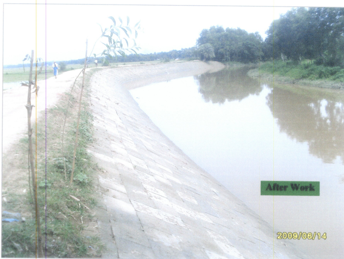
Contract No. BWDB-COM-04: Right bank of Salda river at Nishchintapur, Upazilla : Kasba, District: Brahmanbaria.
