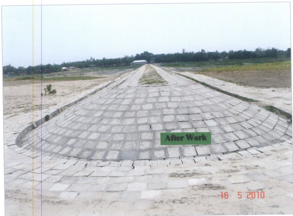
Contract No. BWDB-RAJ-01: Extension & Rehabilitation of spur at Hasimpur bazar, Upazila: Kumarkhali, District: Kustia.
