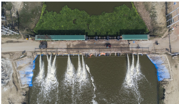
Figure 5: Pumping for removing waterlogging at Bhabadah Regulator
