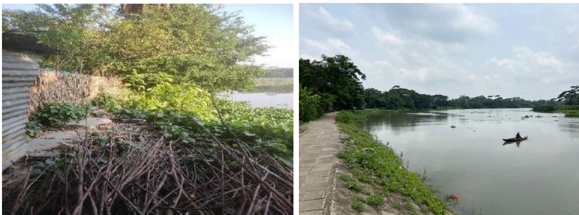
Figure III-2 Erosion at Chitulia river. Source: TA consultants
